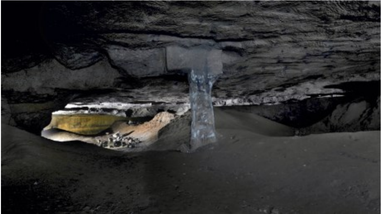
Fig. 9 Stabilising pillar in the chamber of the stone quarry in Kysihýbel (photo by E. Lužina)
