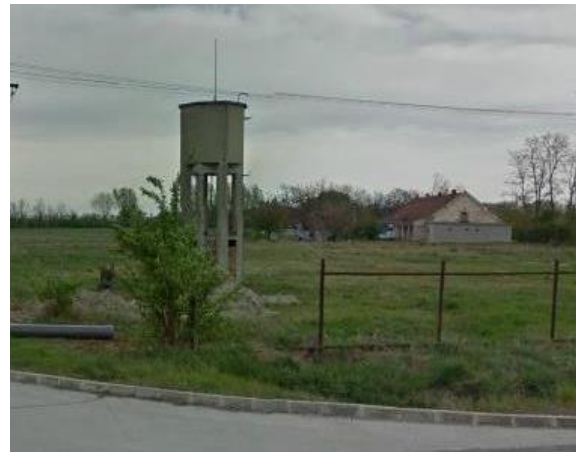
Fig. 6 Water tower and the workers' houses in Jurajov Dvor grange.
