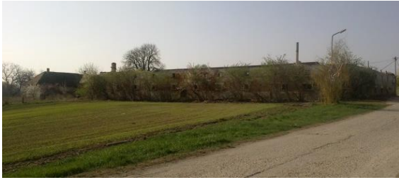
Fig. 5 Damaged buildings in Tárnok grange
