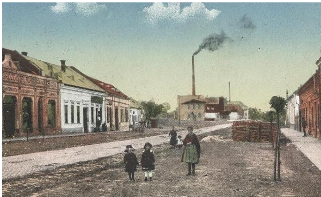
Fig. 6 The agricultural machine factory on the Stúrovo square. Factory building is demolished
