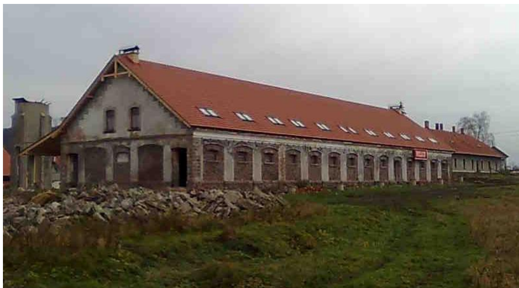
Fig. 9 Farm buildings and stall in Víglaš, part Pstruša. Now are rebuilt by roadhouse with a restaurant and a guesthouse.
