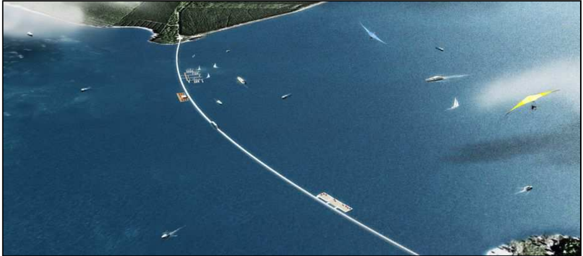
Fig. 10 Floating pontoon in Lake Sedlitz [1,2]
