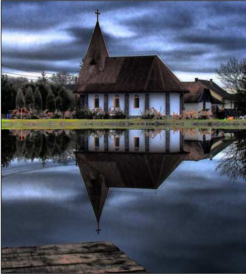
Fig. 6 One of the 3 churches in Bozsva, Source: http://www.panoramio.com/photo/20389937
